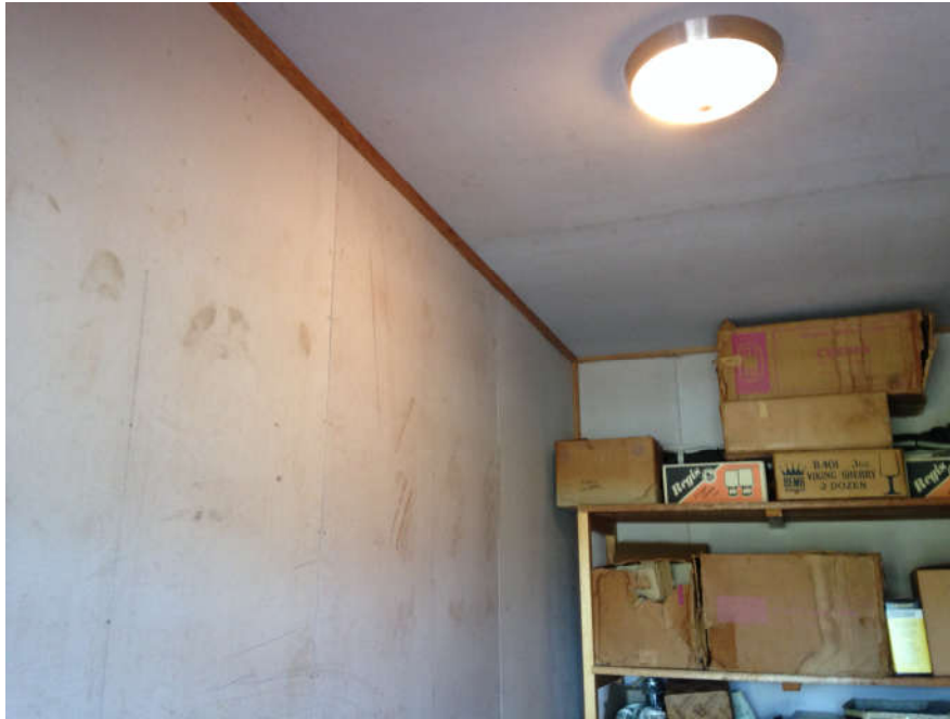
Store room western end unpainted asbestos sheeting
