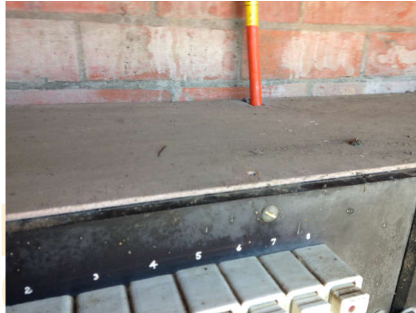
Asbestos cement sheet lining electrical backing boards
