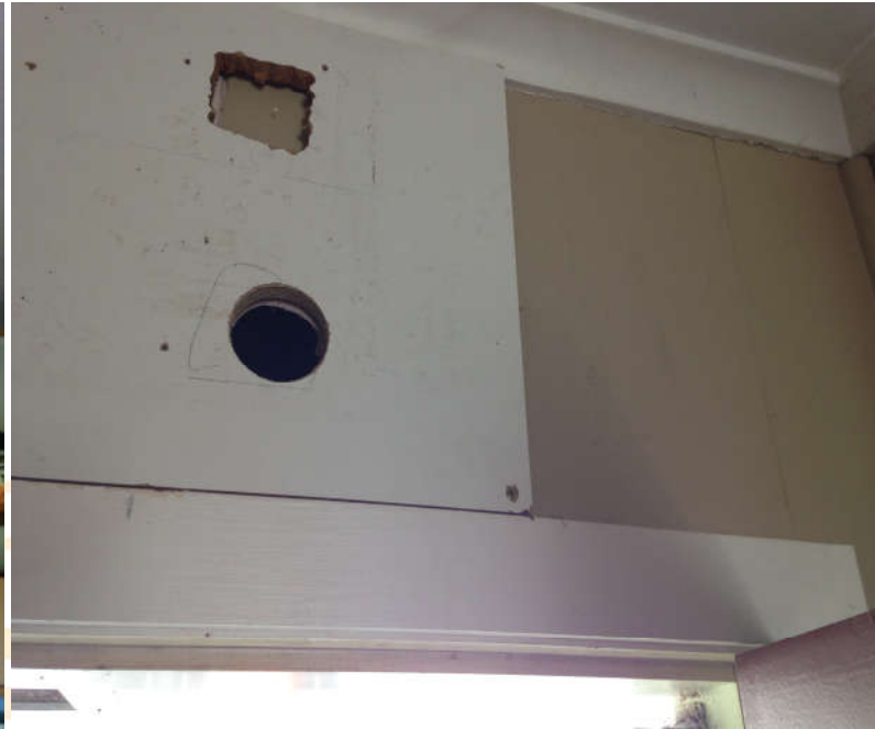
Motel unit #14 with air conditioner removed exposing asbestos sheet
