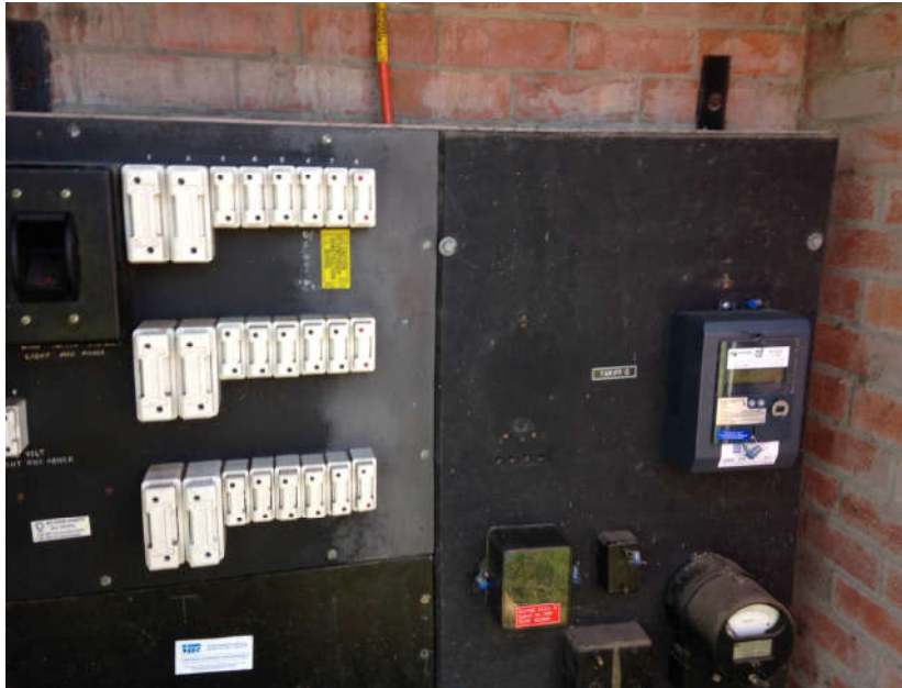
Zelemite asbestos electrical backing boards NOTE: Fuses may contain asbestos
