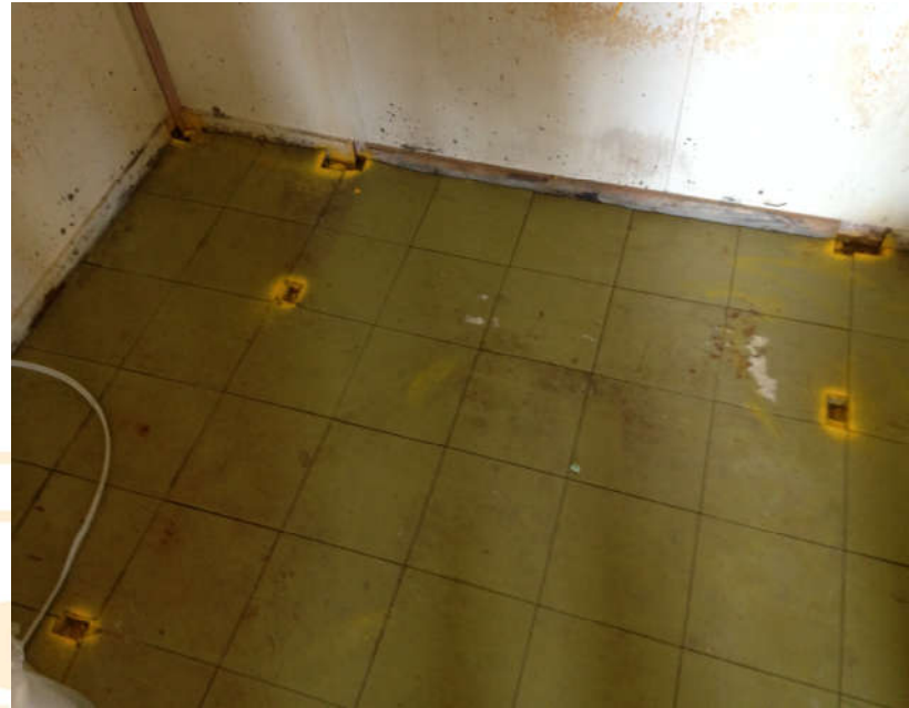
Asbestos vinyl tiles kitchen store penetrations sealed with paint REMOVED 2017
