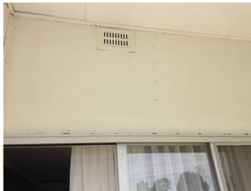
Wall infills above north windows all units – asbestos cement sheet TO BE REMOVED
