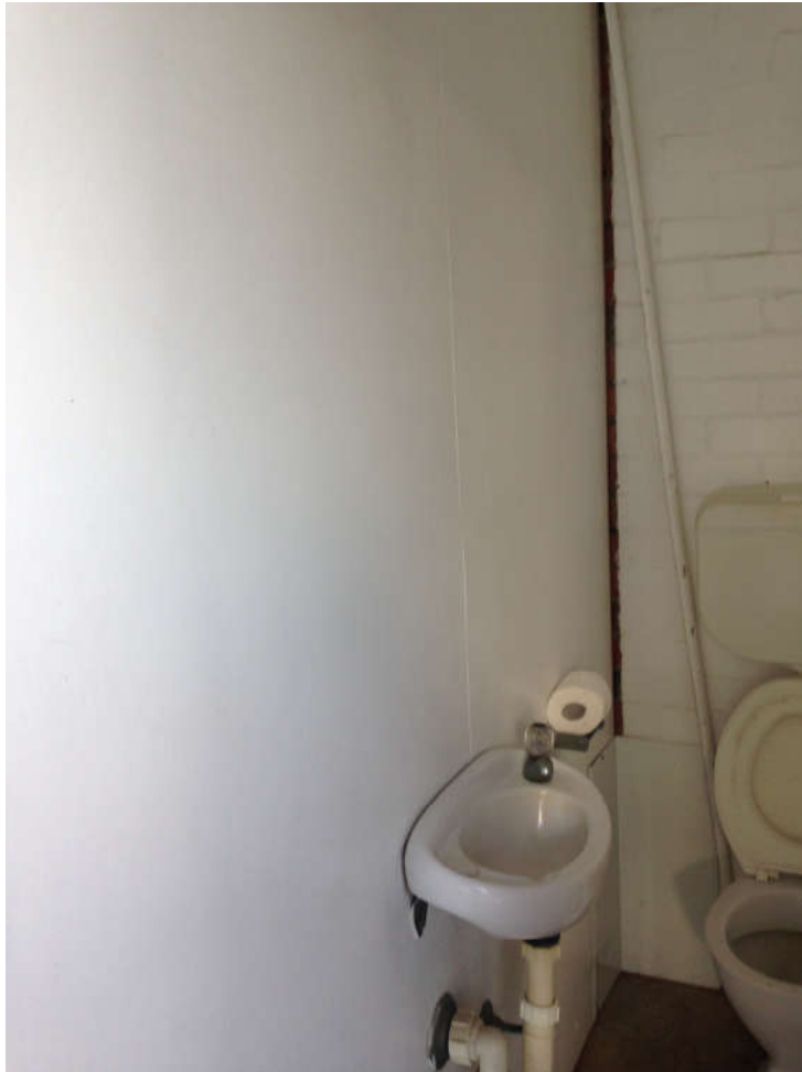
Staff toilet asbestos wall lining
