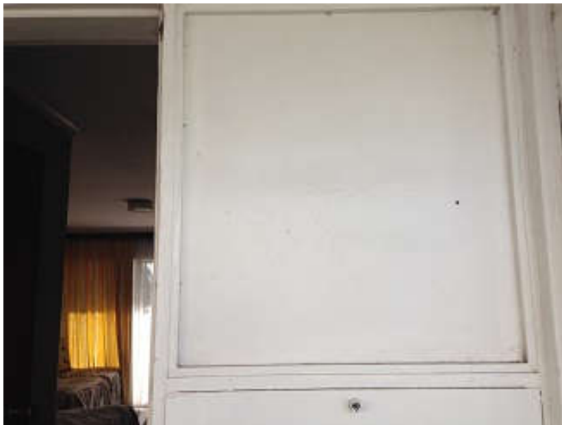
Wall infills above Motel unit server openings – asbestos cement sheet TO BE REMOVED
