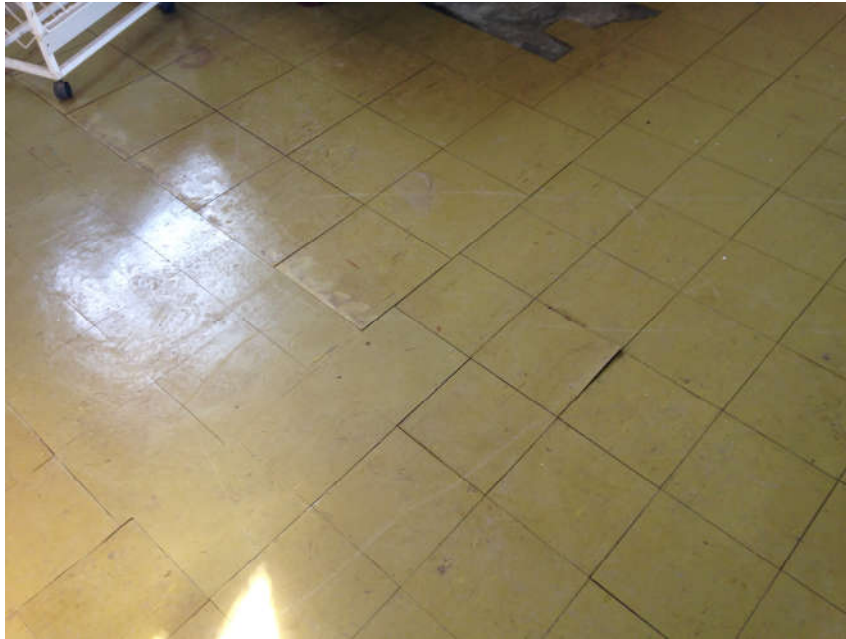
Asbestos vinyl tiles kitchen REMOVED 2017
